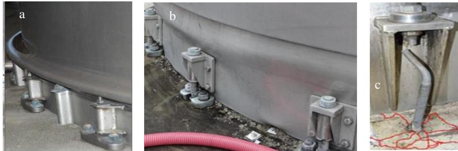
Figure. 5 – Reported damage in Kaikoura earthquake; (a, b) Barrel buckling; (c) Rod rupturing [14]
