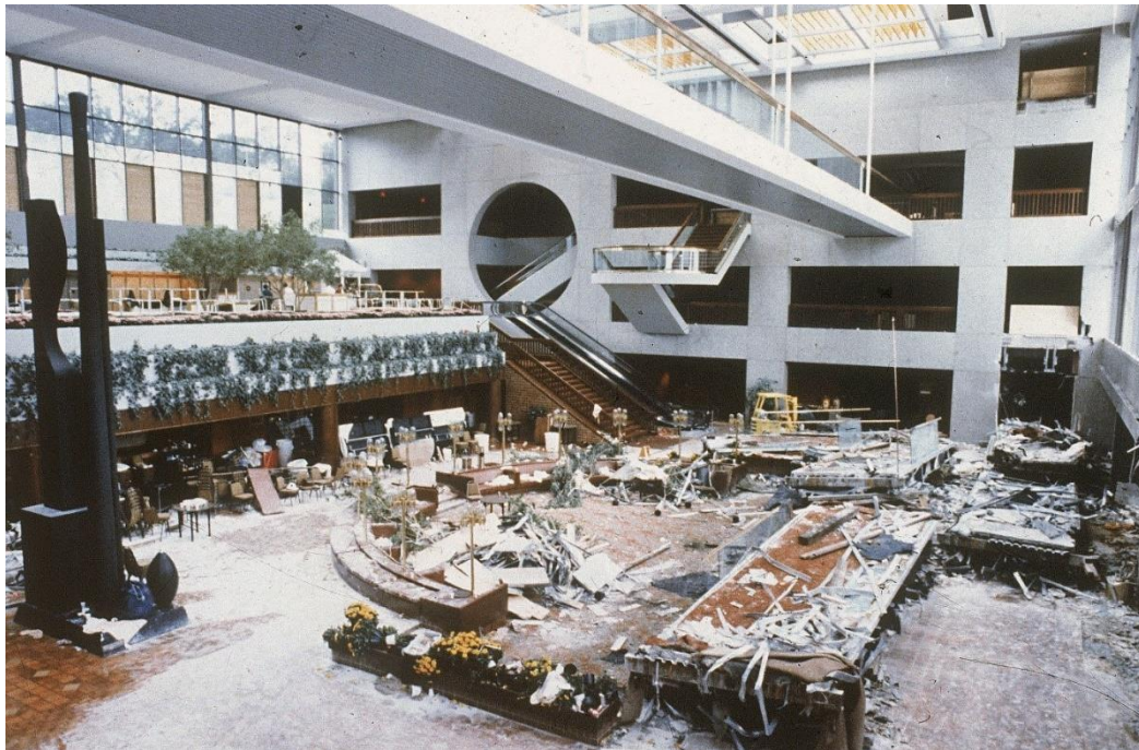
Figure 2 – The collapsed walkway ( https://timeline.com/hyatt-regency-skywalk-failure-8240bff34fa6?gi=4582a0896730 )
